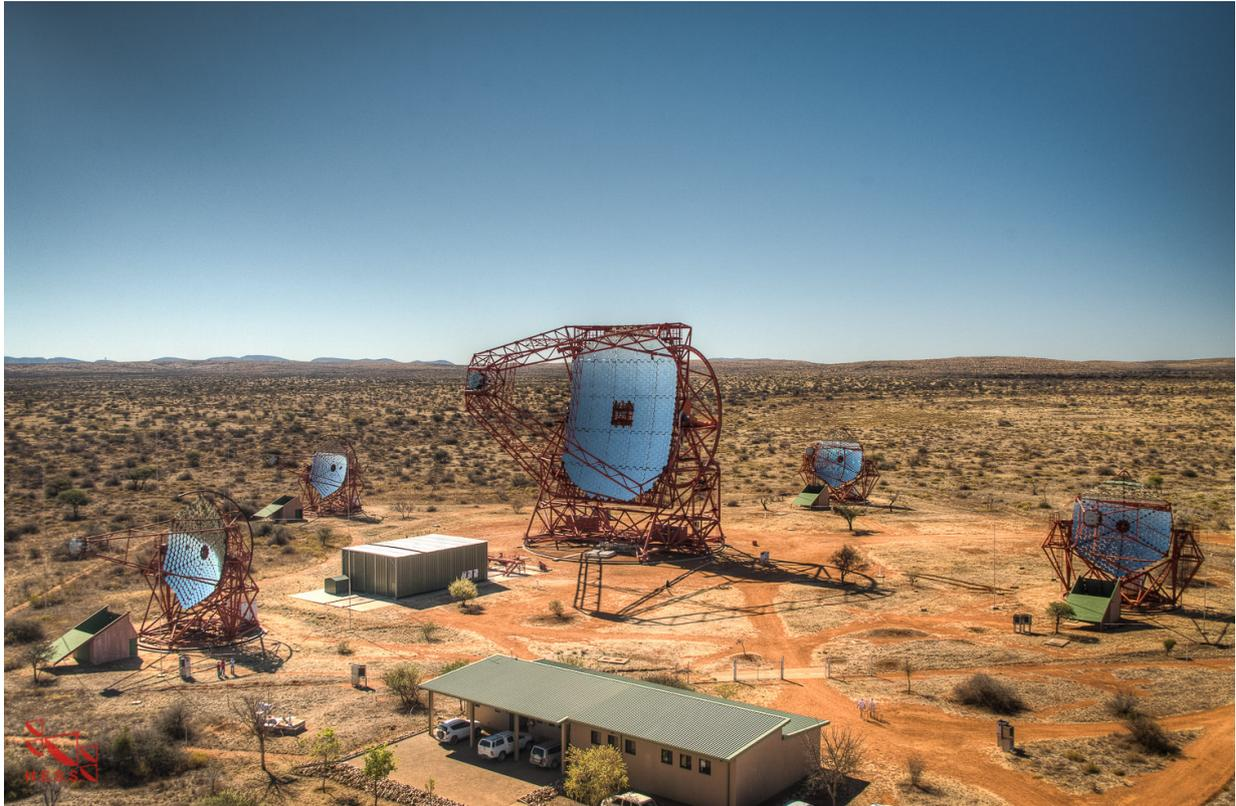
**Figure 3.2:** Aerial view of the full HESS-II array. In front of every telescope is a camera shelter, where the camera is parked during time of non operation. At the bottom of the image is building with the control rooms and the mechanic's and electrical workshops. Image credit: Christian Föhr.
