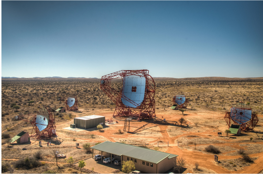
Figure 2.9: Photograph of the layout of the H.E.S.S. telescope array. The four small CT1-4 telescopes are shown forming a square of diameter 120 m with CT5 in the middle of it. A building is visible in the foreground. This building houses the array operation site, the data acquisition system, and the trigger. Credits: Christian Föhr.
